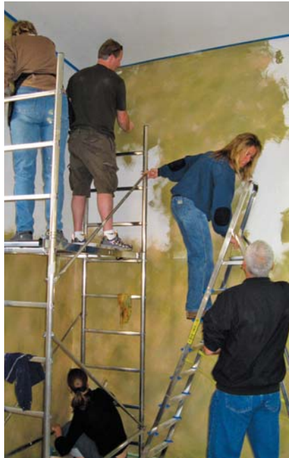
The group does a lime wash.
