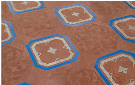
The floor in progress.
