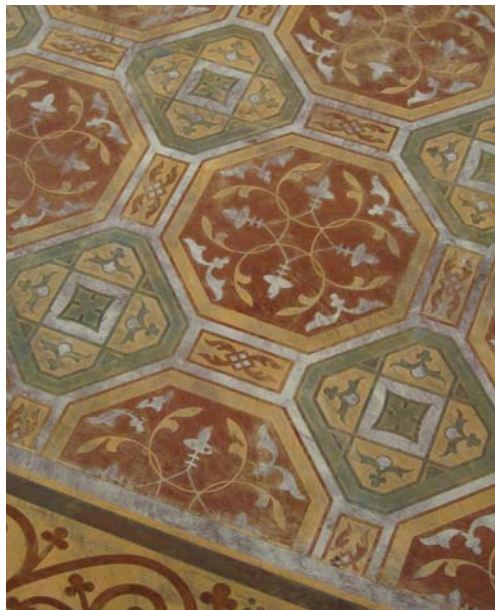
The finished Italian floor.
