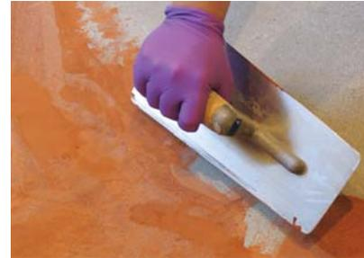
Two thin layers of Florentine Clay were first applied as a base for the center panel of the Chavall carpet. SkimStone is ideally mixed to a thin, almost paint-like, consistency. Simply pour out about a cup at a time and trowel using a Venetian trowel. The material needs to be pulled very tight and thin, so keep the angle of the trowel up and use a good amount of pressure.
