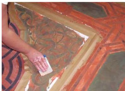
The final detail layer of design is filled in. Here a layer of Winter Olive is applied over a base layer of Florentine Clay to achieve the same shade of green as in the center panel.
