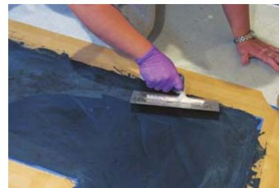
Next the border area is taped off and troweled with two layers of Rainy Day Blue. Use the low tack blue tape (3M orange core) designed for faux painting when taping off edges and areas. Wide paper tape was added to protect the surrounding areas.
