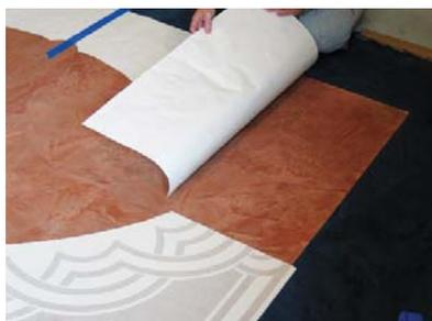
The Concrete Carpet patterns are easily laid out, as they are designed to fit together like puzzle pieces. It's best to have two sets of hands when working with larger patterns, but simply read and follow the enclosed instructions for easy installation.
