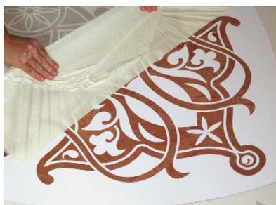
Once the adhesive Modellos are burnished in place, the transfer tape is removed. The transfer tape can be dampened with a large wrung out sponge to loosen its adhesive for easy removal.
