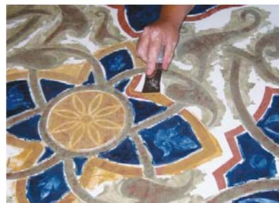
Additional colors are applied in other areas using the Faux Finger tools. The basic technique is to "blade" the colors in using short staccato strokes. Changing directions with your hands will add nice movement and texture, even in smaller areas.
