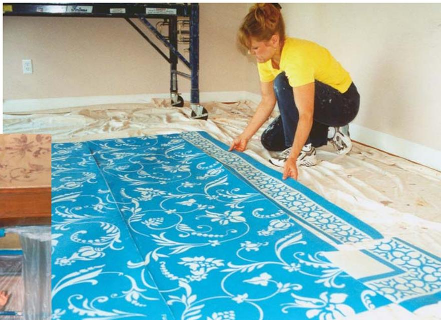
**PROJECT A.** Above: Joanie double-checks the alignment and layout for multiple design “tiles” for a large ceiling project. Below: Once the all-over center pattern has been painted in, the custom fit border pattern is installed. The border pattern was designed and sized to perfectly frame the center panel.
