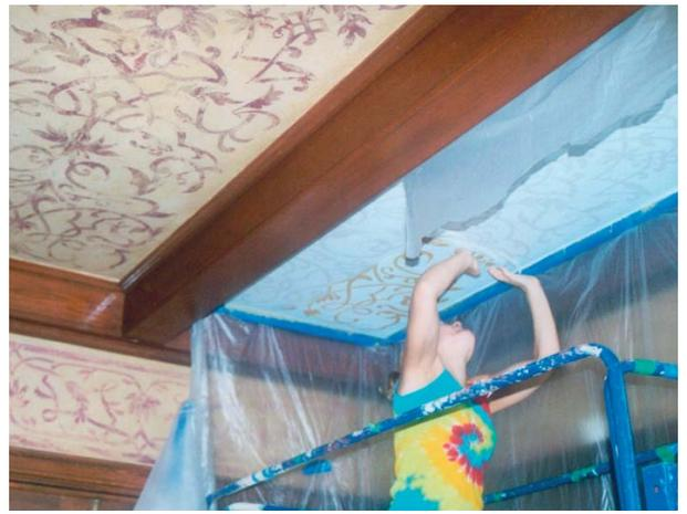
**PROJECT B.** With the Modello burnished in place, the Transfer Tape is pulled off to reveal the pattern that is now ready for embossing. Here, several colors of Lusterstone were “bladed” through the pattern on both the ceiling and companion soffit border.
