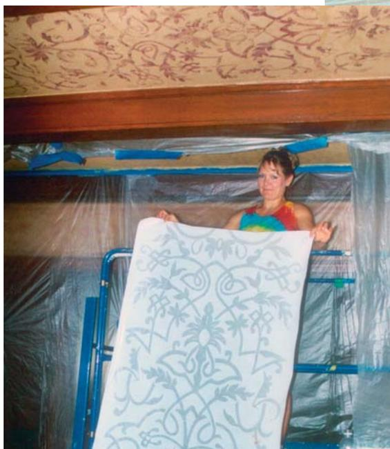
**PROJECT B.** A small panel design was greatly enlarged and repeated to create long, custom panels to run between wooden beams. Joanie’s assistant, Diane, demonstrates the grand scale of the pattern that was easily smoothed into place by two sets of hands. Once one end is secured in place, one artist pulls the Modello taught from the other end while the other smooths it into place from one end to the other.
