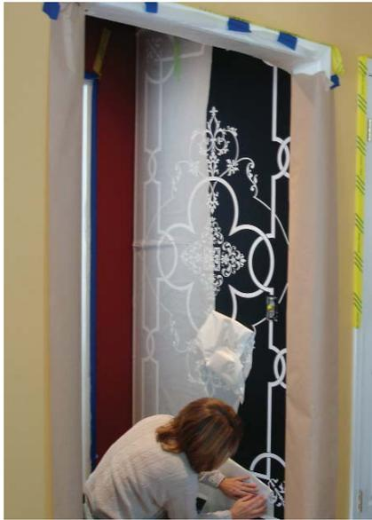
**PROJECT C.** Here a panel design is installed in an entryway over a black basecoat. This photo shows the transfer tape being removed. This particular Modello is a “negative” or “resist” design that is used to create an inlaid pattern.
