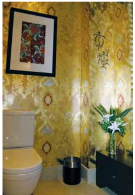
Metallic plasters, glazes, metal leaf and metallic foils were used for most of the surface finishes.
